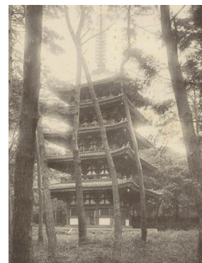
Daigoji Gojyū no tō (Daigoji, pagode) [Afb. 12], Kyoto, foto uit Kenchiku Kōgei Gakan, Kyoto, Kenchiku kōgei kyōkai, 1/12 (januari 1913), frame 3/19. National Diet Library Digital Collection
